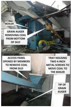
Photo 5. Grain auger used to remove coal before explosion. *(NIOSH photo)*
