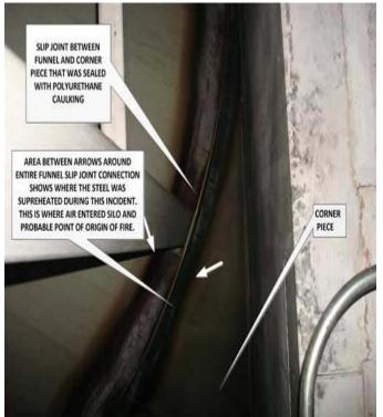
Photo 3. Shows lines of demarcation where fire was burning inside silo around the slip joint between the funnel and the corner pieces. (NIOSH photo.)
