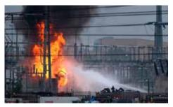
After receiving word from Con Edison, firefighters began applying Purple K to the transformer from two lines, but it kept re-igniting. So they applied foam and Purple K, but it continued to reignite. After 1 1/2 hours, they tried F-500 Encapsulator Agent, mixed with water at 3% through a single hand line. Since F-500 EA has the ability to cool the massive metal transformer and encapsulate the oil, F-500 EA extinguished the fire in less than two minutes.
