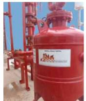
HCT engineers and packages Concentrate Control Supply (CCS) systems to precisely proportion F-500 Encapsulator Agent into the fire suppression system water stream. These systems typically include a bladder tank or other water-driven proportioning system, sized to maximize sprinkler and spray mist system effectiveness.
